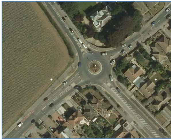
Figure 16 - A256 / A255 Dane Court Roundabout
