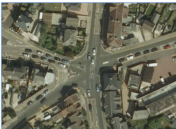
Figure 18 – Victoria Traffic Signals
